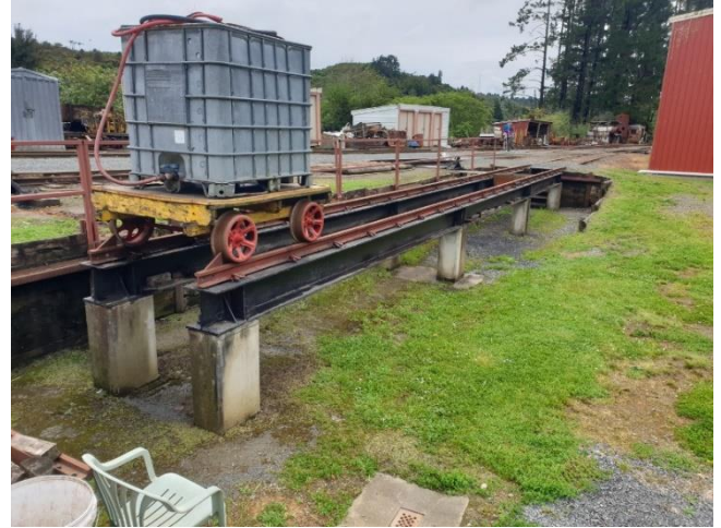
Right: Inspection pit.
